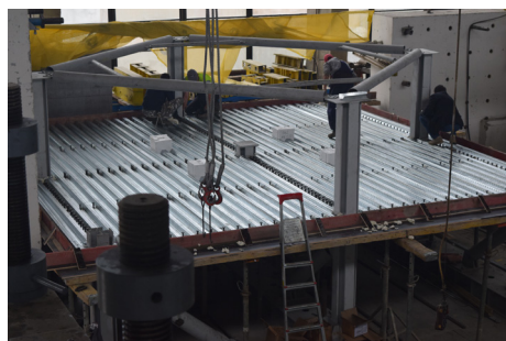
Fig. 6. Composite slab system during construction
